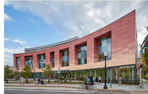
Front elevation, King Open School © Robert Benson Photography
